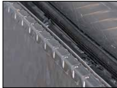
Fully concealed aluminum continuous hinge.
